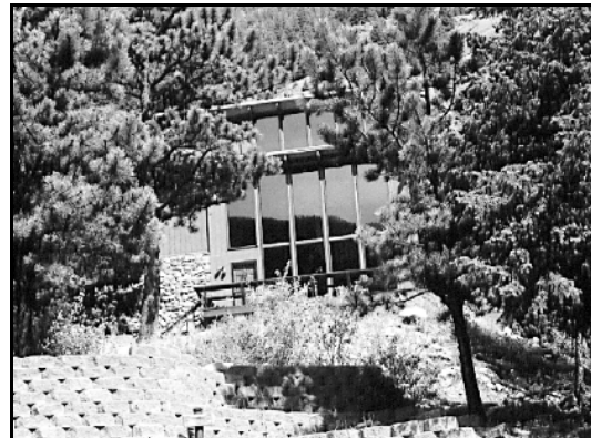
Large areas of glass in exterior walls that may allow "spill-over" of interior light sources, resulting in nighttime glare, should be avoided.
