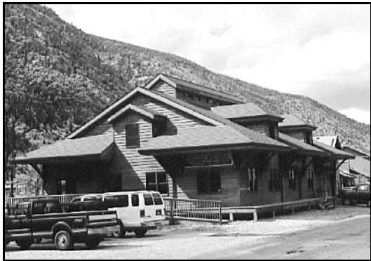
Long ridgelines parallel to the street shall be broken by dormers, setbacks or in some other fashion.
