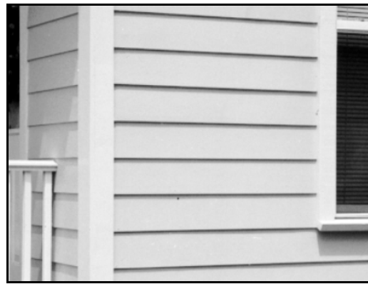
Synthetic materials, such as this composite cement board, may be considered if they appear similar character and detailing to traditional building materials.
