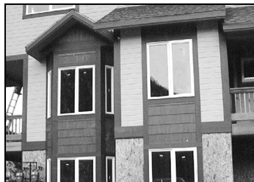
For larger buildings and projects on large parcels, consider a combination of appropriate materials as a means to reduce the apparent size of the project.
